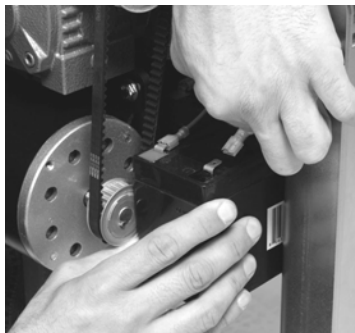
Reconnect the wires onto the replacement batteries.
