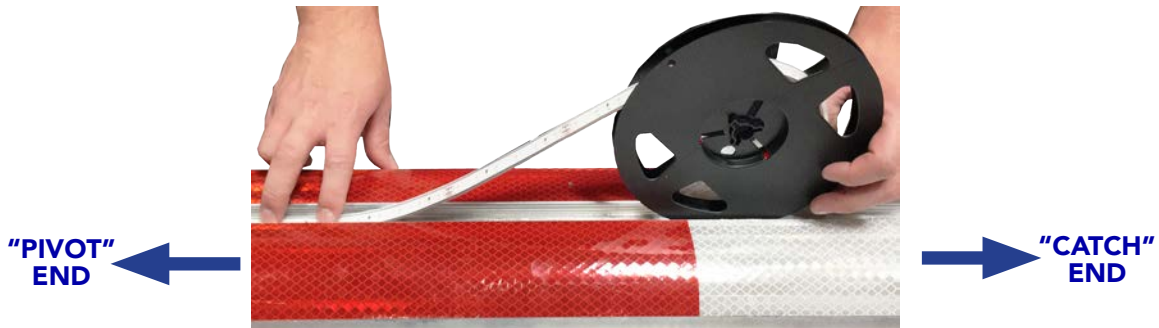
IMAGE 6-2: LAYING OUT LED STRIP IN LED CHANNEL
