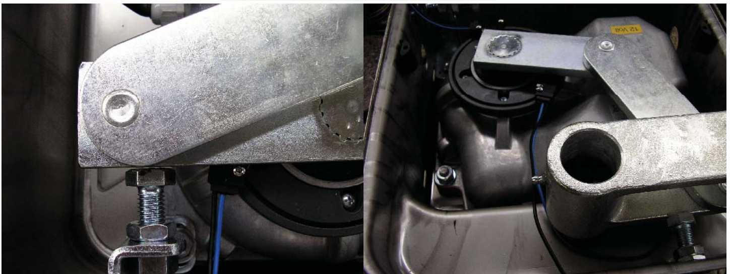
Move arm to close stop and install close limit switch with supplied screws so that switch is activated..
