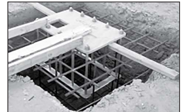
Aligning Rebar & Anchor Cage
