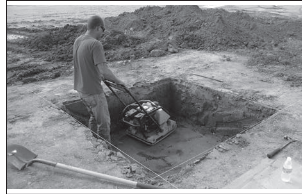
Soil Density compacted to 95% per ASTM-698
