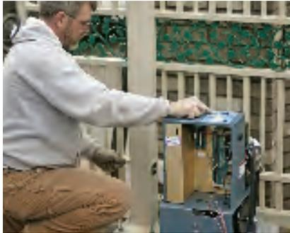
**5a.** With your **gloved** hand keep feeding cable on drum. Carefully add cable by pressing and releasing the Open button, keeping cable wrapped tightly together.
