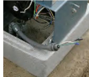
2. Feed AC wires through pad into conduit.
