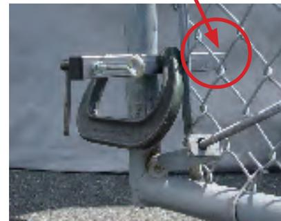
**7. Cut leading edge tubular bracket in place and permanently weld or U-bolt to gate.** Be certain to mount on inside of gate frame to reduce protrusion.
