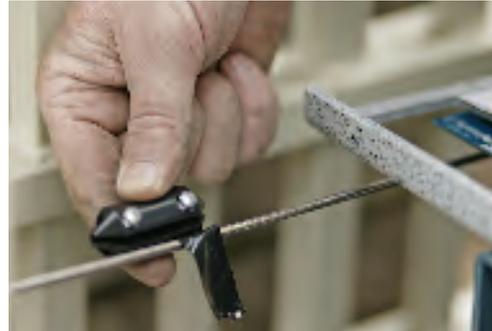
3. After you've marked the cable, push OPEN or CLOSE on SlideWinder's membrane switch, moving the cable mark so it's visible, away from the drum. When it is visible, push STOP. This installer used a piece of electrical tape to indicate Pickle placement. Remove tape when you've attached and secured the Pickle.
