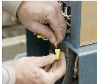
4. Attach black, green and white wires with wire nuts or crimp bonds.
